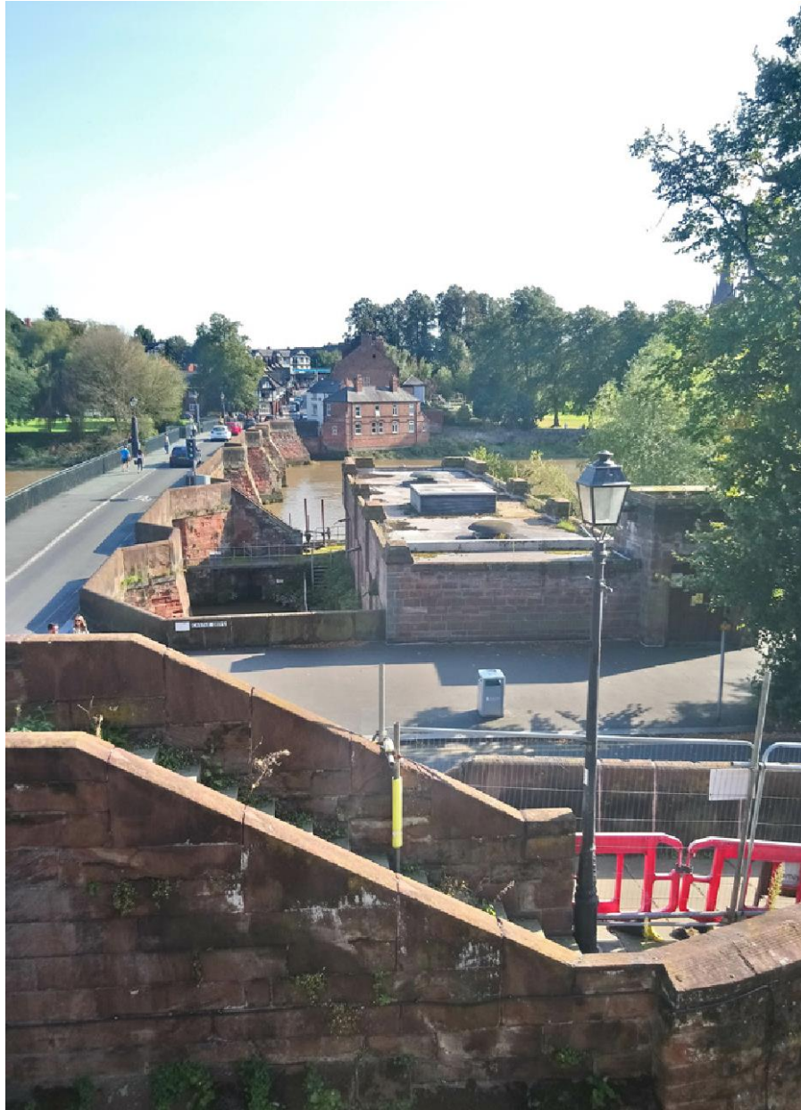
The Hydro Electric Station with the City Walls in the foreground
